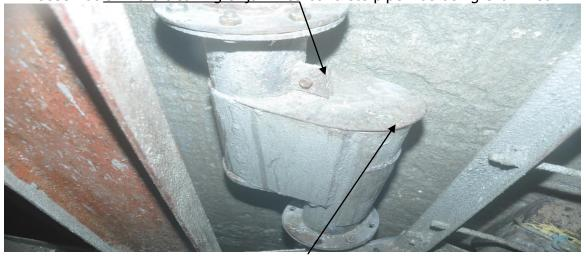
Open flap from where slurry and water splashed when jammed pipe abruptly opened
