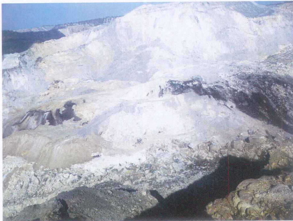
Photograph showing profile of dump slide.
