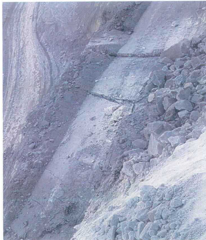
Crack on OB dump haul road.
