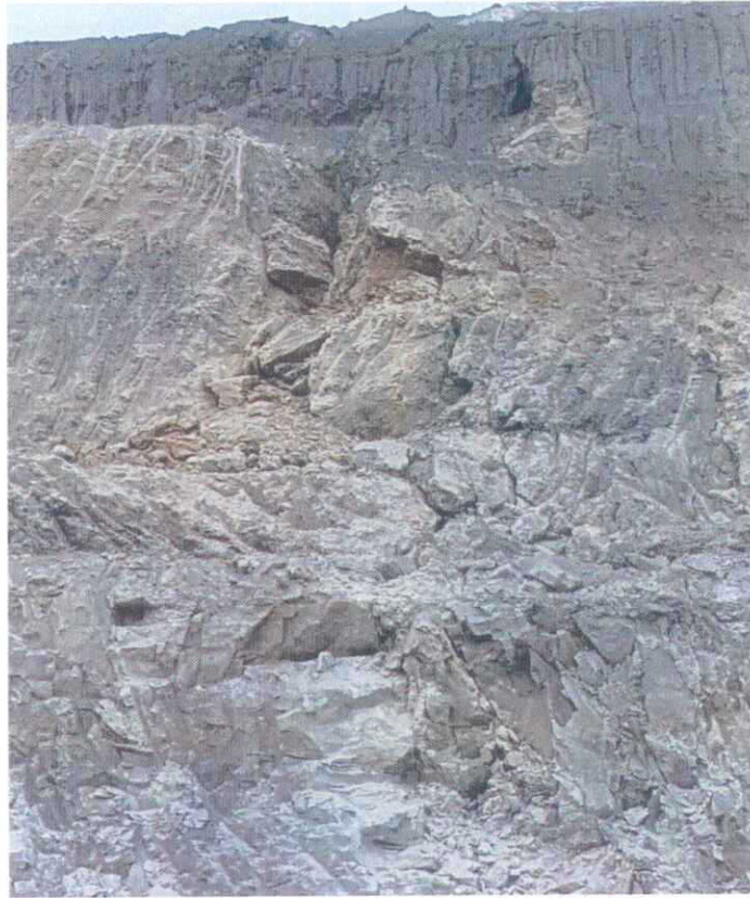
Vertical Crack in in-situ OB bench
