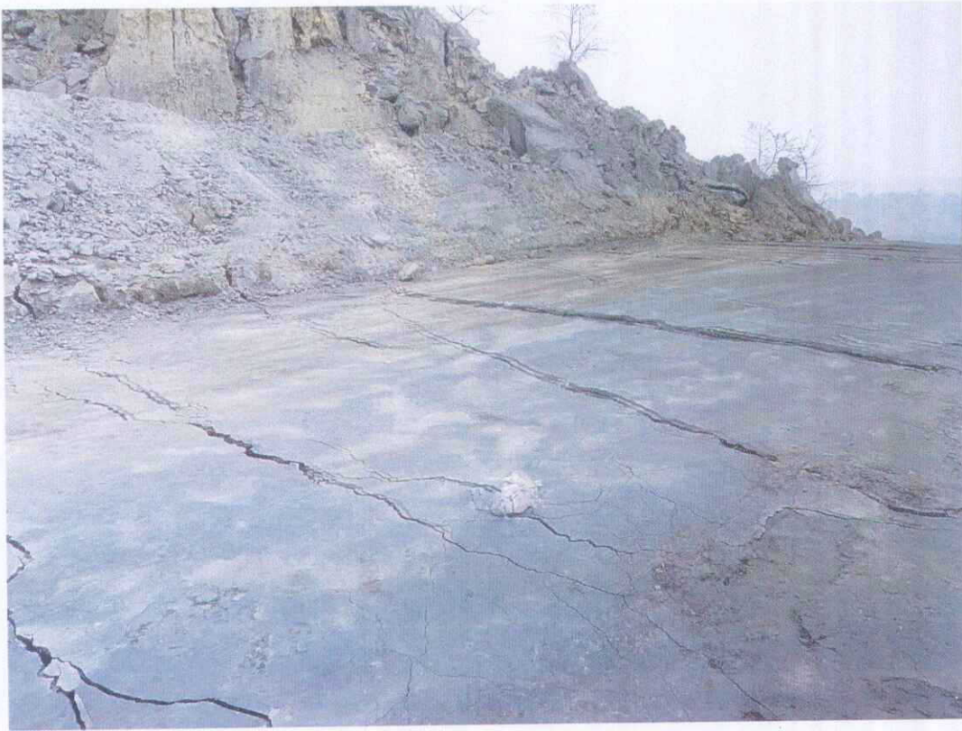
Photograph of crack in OB dump haul road.
