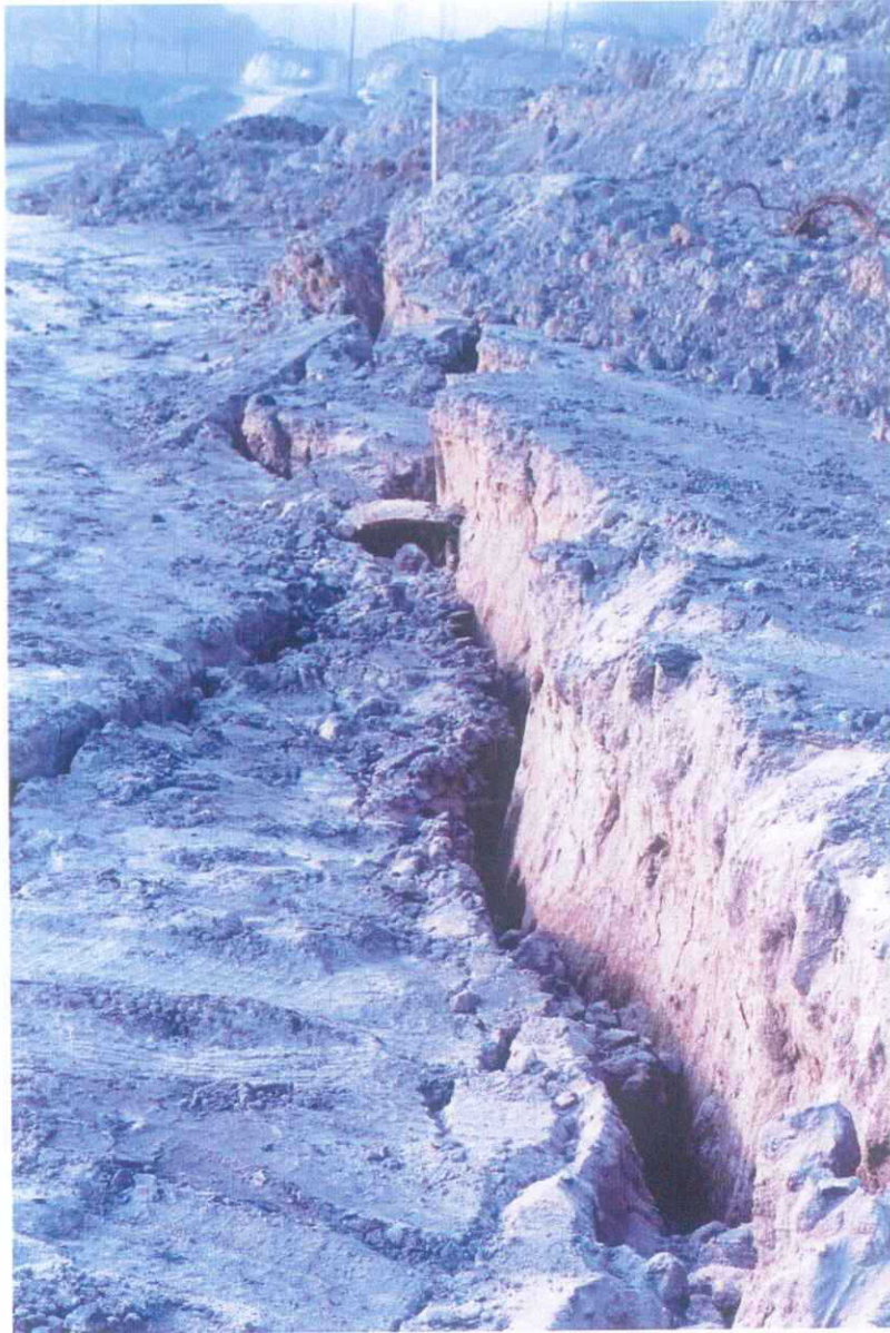
Photograph showing prominent crack & subsiding of OB.
